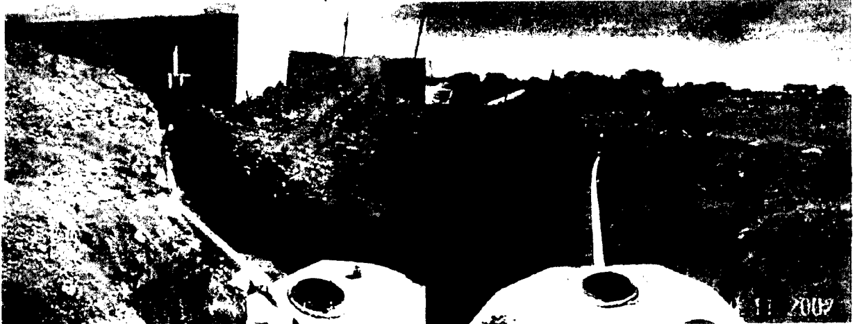
Tank to House looking South
