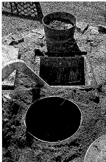
1250 gallon tank 2 Compartment
