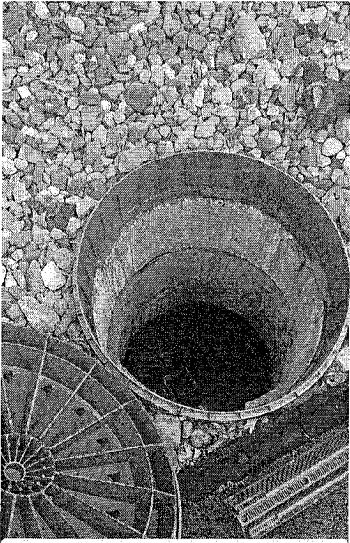
System has filter in the green lid. That needs to be cleaned every year
